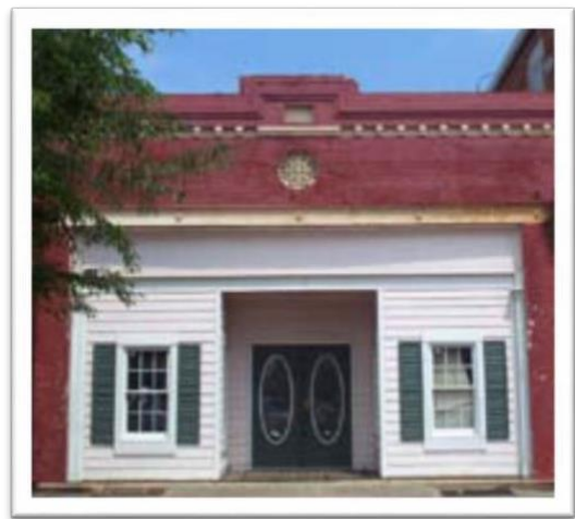
Figure 3: Inappropriate treatment of a historic storefront, including the vinyl siding, residential style entry doors, and residential style windows with shutters.*
